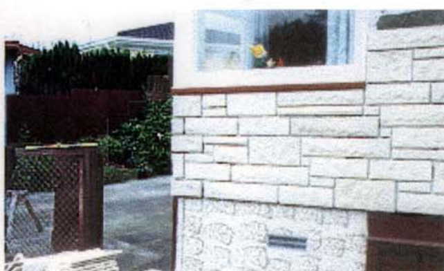
The setting can be commenced from the bottom, top and center
