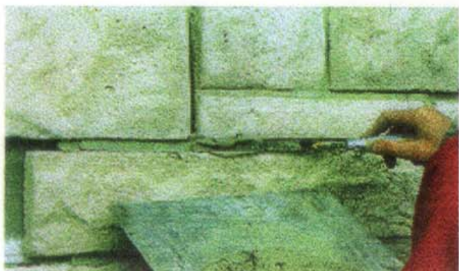
The top of space should be approx 5-10 mm under surface
