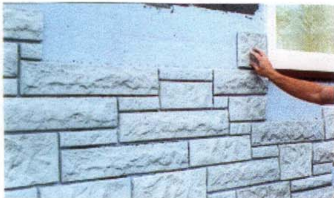
Horizontal line to assist the perfect and neat installation
