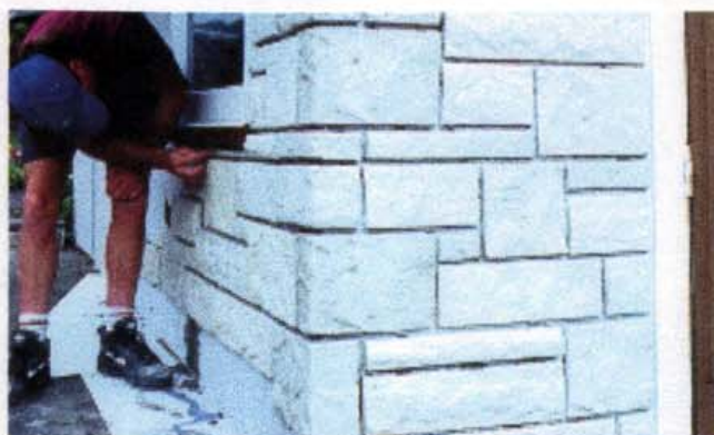
The installation starts from the corner
