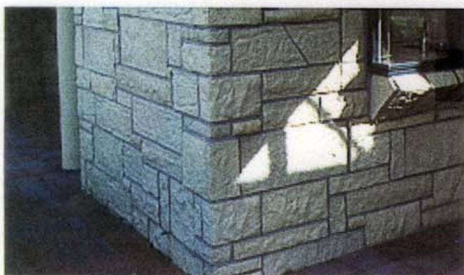
The stone is easy to cut by using cutting machine
