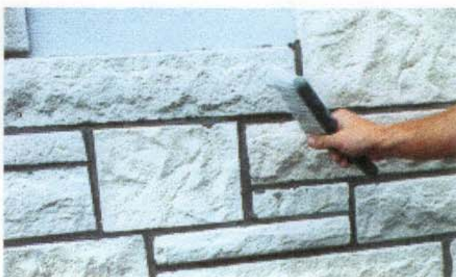
Clean the surface of stone by using nylon brush
